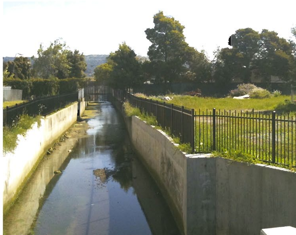
View of concrete culvert to the north
