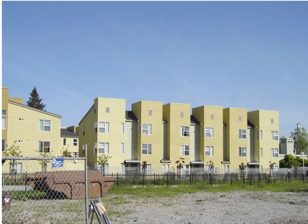
Detail of cement plaster bays and horizontal siding
