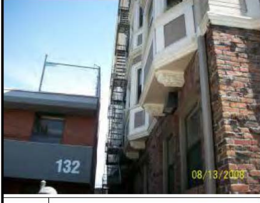
3. Partial view of west facade
