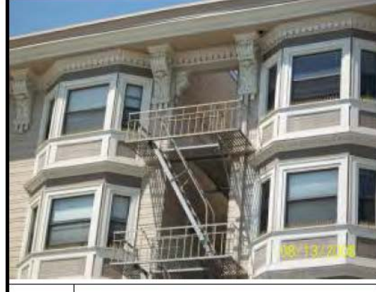
6. Detail of windows and fire escapes
