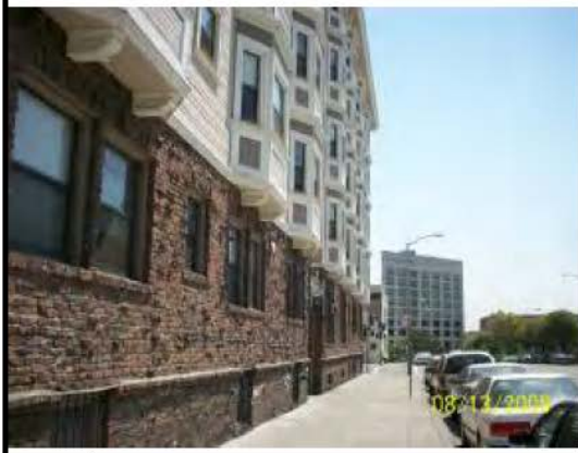
2. View north from southwest corner of the subject property
