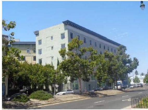
2. East façade of building
