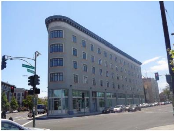
1. View of building façade looking south
